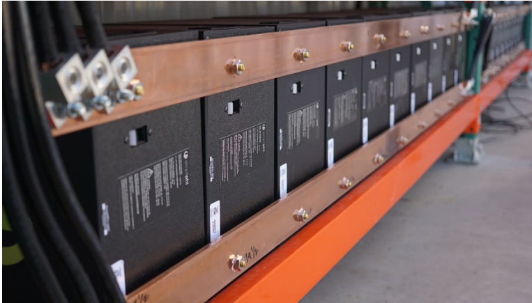
Figure 4.0 – Three PHI Batteries Paralleled Using Direct Bussing
